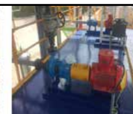
ULP & JetA1 Pump/Motor
