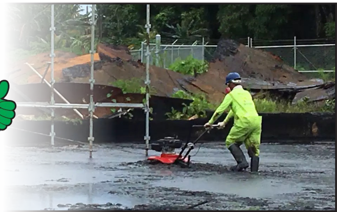
C4Life team member aerating the sludge; remnants of Tanks 2 and 3 visible in the background.
