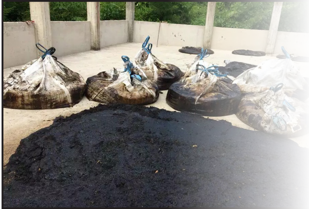
An estimated 290 cubic yards of sludge-contaminated soil was extracted from Tank 1 and is currently undergoing the bio-remediation treatment.
